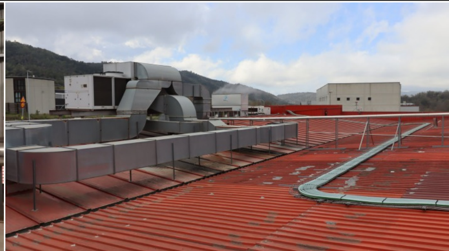
Sostre nau principal
