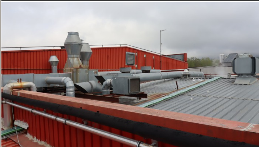
Sostre nau principal
